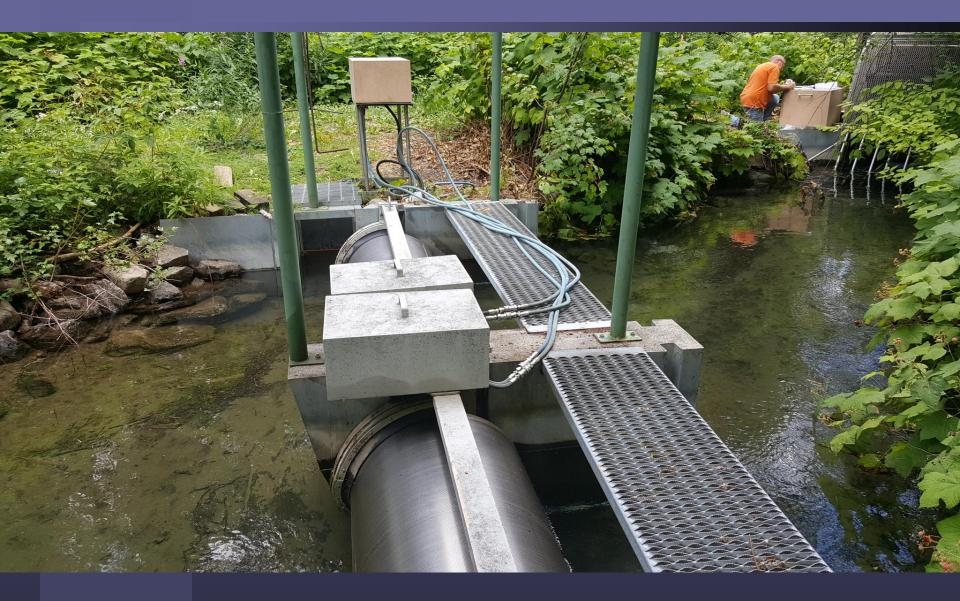
During a past Fish Screen & Passage Workshop in Idaho. The tour took us to a site that had multiple drum screens. They had two drum screens being driven by one paddlewheel. There was the ability to isolate the paddle wheel for maintenance without shutting the system down.
